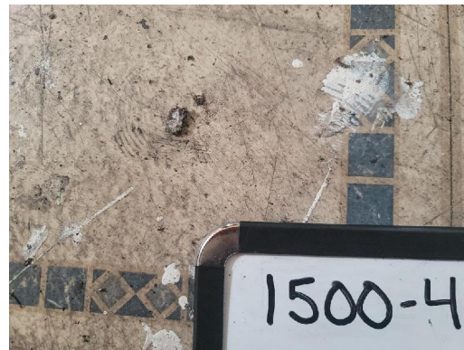
1500-4 12"x12" Floor Tile/Adhesive Interior Southwest Bedroom
