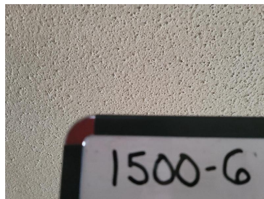
1500-6 Popcorn Texture/White (2% Chrysotile) Typical Interior Ceilings/Appx. 800 sf
