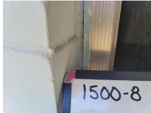
1500-8 Glazing/Off-White (2% Chrysotile) Typical Exterior Windows
