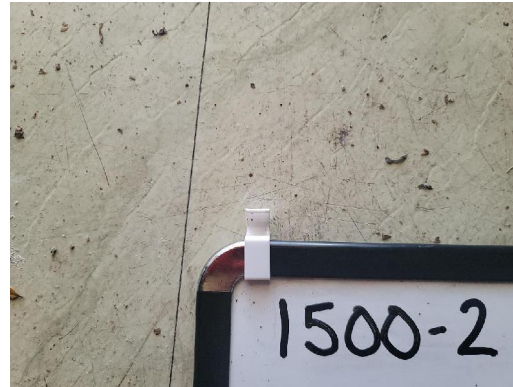
1500-2 12"x12" Floor Tile/Adhesive Typical Interior (Top Layer)
