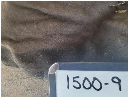
1500-9 Roof Felt Typical Exterior Roof
