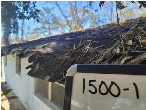
1500-1 Asphalt Shingle/Tar Typical Exterior Roof
